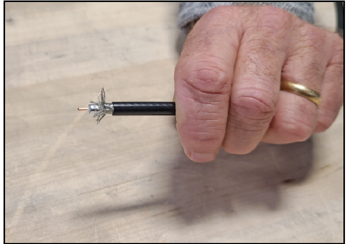
Figure 51: Flaring the Braid
