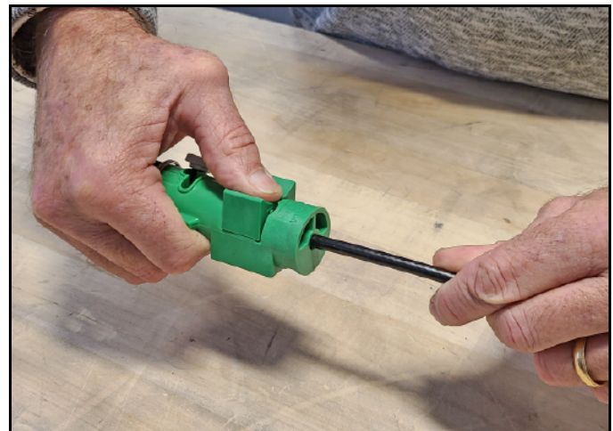
Figure 47: Stripping the End to Expose the Center Conductor
