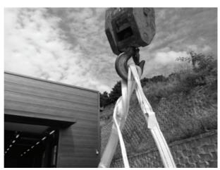
B. Secure the strap tightly as shown left for a safe removal.
