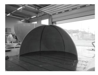
A. The assembly of the upper radome panels should now be completed, using the M6 x 35 bolts supplied.
