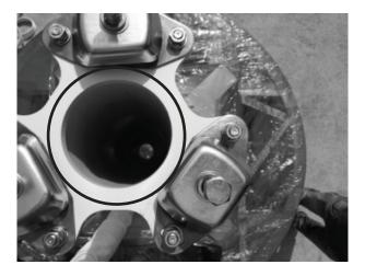
C. The cables need to be inserted through the center of the pedestal support as indicated
