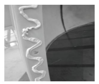
B. Apply silicon (Sikaflex-291) to side of radome panels before fastening bolts.
