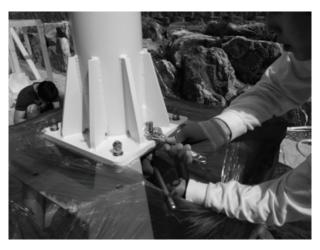
D. Secure the lower pedestal to the base frame with the 8 M12 x 60 bolts supplied. Lock the bolts by installing double nuts onto the bolts. Make sure to apply Loctite 262 to the bolts to securely tighten the assembly.
