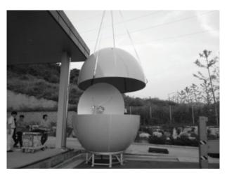
D. Apply silicon to the top lip of the lower section of the radome then slowly place the upper radome on to the lower radome half. Slowly place the upper radome on top of the lower radome assembly.
