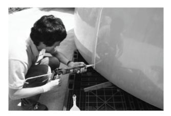
A. Apply the silicon from the outside between the radome panels.
