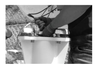
D. Place the cables through the center hole of the Post as shown in C.
