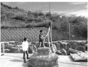
E. Lower the base frame onto the floor and remove the lifting assembly.
