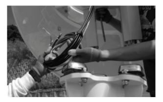
A. Locate the power and RF cables as shown.
