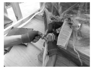
C. After applying buckle ropes to all 4 corners, attach lifting strap to buckle ropes.
