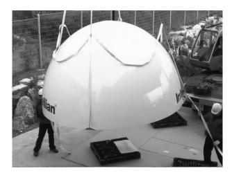
B. Connect the lifting strap to the radome.
