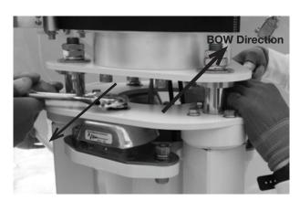
B. Insert the 3 M16 x 40 bolts to secure the antenna assembly to the pedestal. Make sure to apply Loctite 262 to securely tighten the assembly.
