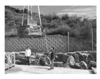
D. Very slowly lift up the base frame and watch as the base frame lifts up to prevent big interference with wooden crate.
