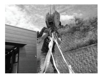
A. Now prepare to attach buckles to base frame in order to lift the base frame from wooden crate.
