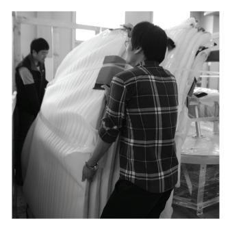
B. Carefully remove the radome panels.
