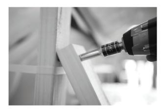
A. Remove the wooden bar that supported radome panels using an Impact Drill.
