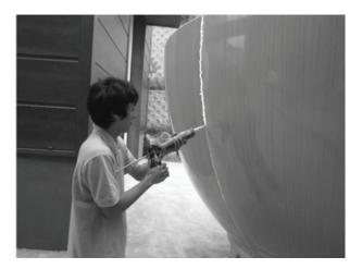
A. Apply the silicon between the radome panels from the outside.
