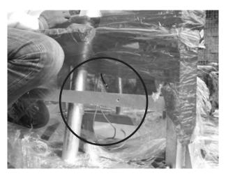
E. Cables should come out of the bottom of the post as shown left.
