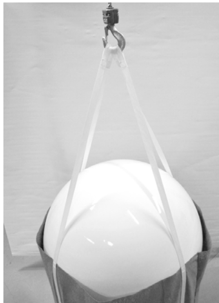
Figure 2-23: ADU installation, 4 lifting straps on crane hook
